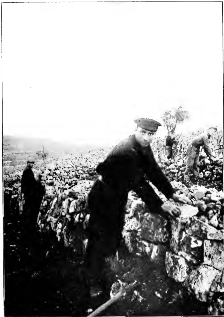
The colonists terrace the hillsides to hold back the soil with stones cleared from the fields, once thought too rocky for cultivation. Many neglected and treeless hills have been utterly denuded of earth by the rains of centuries
